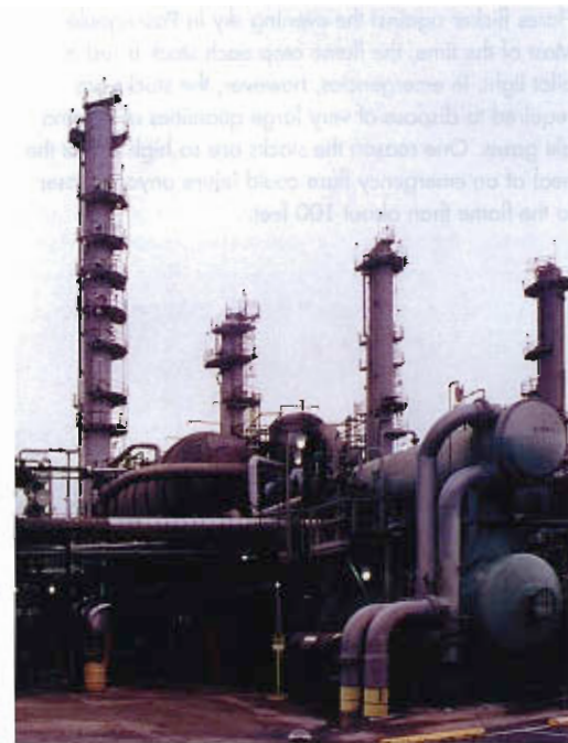
An alkylation plant at Pascagoula (above) also relies on bullet-tank pressure vessels, but in this case they are laid down horizontally; one large tank is visible here behind the smaller drums of a heat exchanger. The unit also includes several tall distillation towers.
