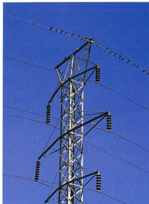
Aerial ground wire ( above ), at the very top of the tower, provides a perch for pigeons, which avoid the high-voltage conductors lower down. But the aerial ground is not put there for the convenience of birdlife; it protects the power conductors from lightning strikes. Another form of lightning protection ( below ) relies on an arrester—the slender rod to the right of the insulator string—to divert voltage surges through the tower and safely into the ground. Arresters are common in substations but rare on power lines; this specimen was photographed in Spartanburg, South Carolina.
