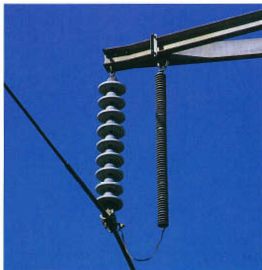
Aerial ground wire ( above ), at the very top of the tower, provides a perch for pigeons, which avoid the high-voltage conductors lower down. But the aerial ground is not put there for the convenience of birdlife; it protects the power conductors from lightning strikes. Another form of lightning protection ( below ) relies on an arrester—the slender rod to the right of the insulator string—to divert voltage surges through the tower and safely into the ground. Arresters are common in substations but rare on power lines; this specimen was photographed in Spartanburg, South Carolina.
