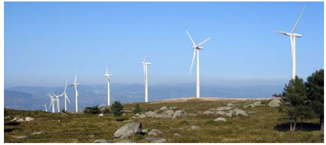
Fig. 16. Wind turbines at a wind farm in Galicia, Spain. Aerodynamic and electrical interaction among turbines on a wind farm can result in energy capture losses. Better modelling and coordinated control of such arrays of multiple turbines can recover some of these losses. Photo from [42].
