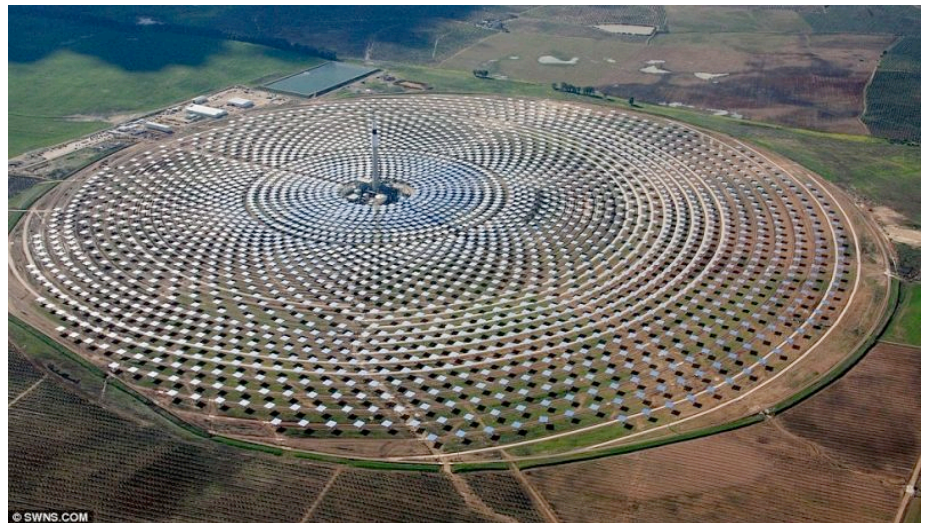
PS20 power tower, Seville, Spain, 1255 mirrors, power up to 20 MW. Operational 2013. Image: SWNS.com.
