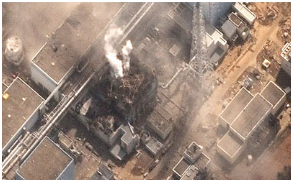
Fukushima power station (Tokyo Elect. Power) Units 1, 2, 6 1971 GE Mark I BWRs
