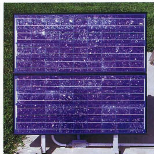
Photovoltaic cells, which generate electricity directly from sunlight, are made of polycrystalline silicon. The array of cells above is installed at Montgomery College in Germantown, Maryland. A detail, below, shows the grain structure of the silicon material and the grid of metallic conductors laid down over it to collect current.
